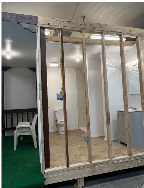
Program participants applied their newly acquired skills to framing and building this fully functioning structure that includes lighting and an operational full bathroom (toilet, shower, and running water).
